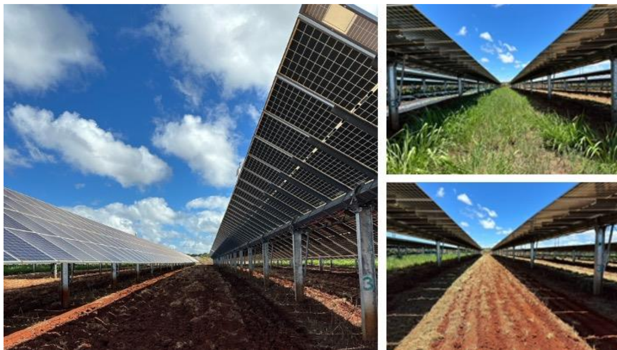
Image 5. Conversion of conventional PV landscape to Agrivoltaic footprint. From left to right: ripped and disked ground ready for amendments and a follow up disking to incorporate the amendments, undisturbed environment in typical photovoltaic landscape of Guinea Grass and wild plants, ripped but not tilled soil preparation.
